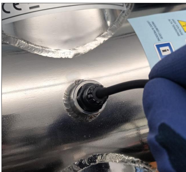
c) Make sure that the sensor element (at the end of the cable) is in contact with the bottom of the bush
