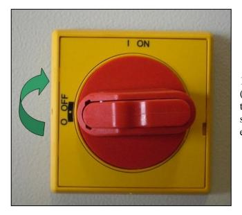
10 Turn the UV system on with the general switch (the lamp will light after few minutes). Do not open the electrical panel without turning off the general switch. We remind you to test the differential switch every month.
