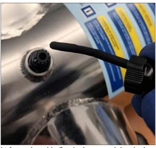
b) Insert the cable first in the cap and then in the cable gland
